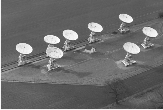
Figure 4. LA from the north-east. The correlator is in the central hut. The railway track, which runs diagonally across the photograph, is approximately east-west. Four antennas are moveable along the track.
